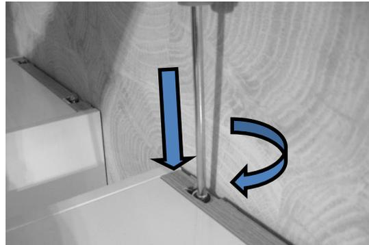
For the height adjustment of column-cabinet, half column-cabinet, mirror with shelf, mirror-cabinets, screw clockwise or screw anti-clockwise as pictures.
