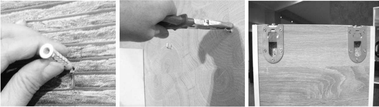
1. For the wall-fixing of column-cabinet, half column-cabinet, mirror-cabinet and mirror with shelf, drill a hole with a twist-drill of diam. mm.8-05/16 following the previous signs, drawn with a pen, insert the dowels inside the holes, then screw with the supplied key-hook.
