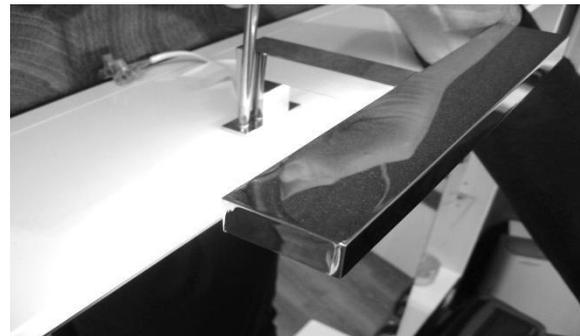
**2.** In case of installation of mirror with shelf or mirror-cabinet, before to hang the element at the wall, connect the electrical installation. Pay attention: before any electrical arrangement, disconnect the main voltage power supply, later connect the cables of the Driver to the main electrical power 220-230V according to electrical polarity.
