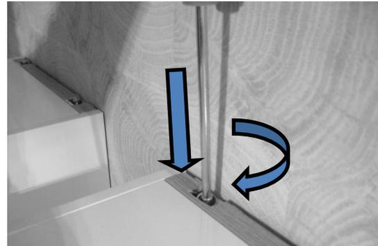
**3.** For the height adjustment of column-cabinet, half column-cabinet, mirror with shelf, mirror-cabinets, screw clockwise or screw anti-clockwise as pictures.
