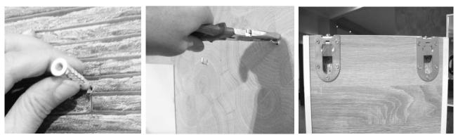
1. For the wall-fixing of column-cabinet, half column-cabinet, mirror-cabinet and mirror with shelf, drill a hole with a twist-drill of diam. mm.8-05/16 following the previous signs, drawn with a pen, insert the dowels inside the holes, then screw with the supplied key-hook.
